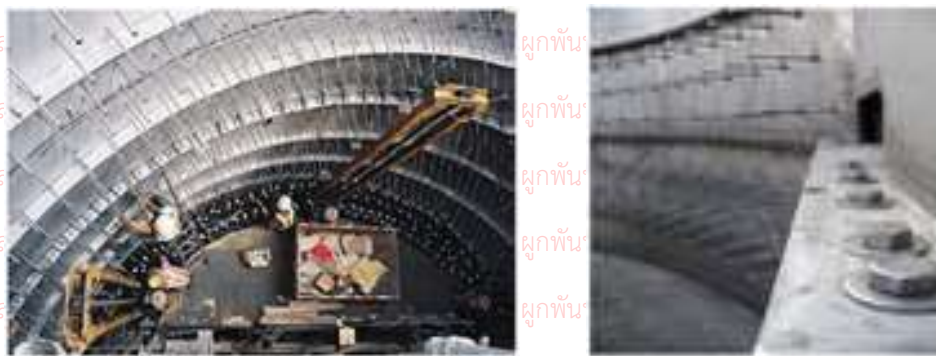
Shear connectors on the inside of a tower segment
