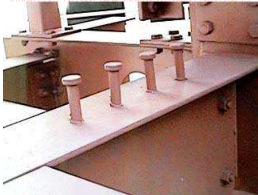
Shear Connectors for Composite Beam
