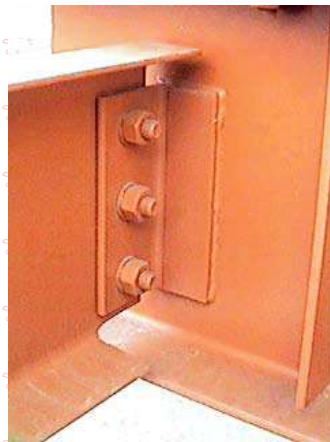
Single Angle Shear Connection
